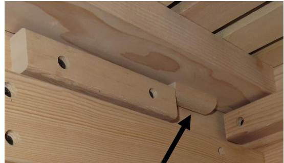
Wood STOP on Underside of BENCH
