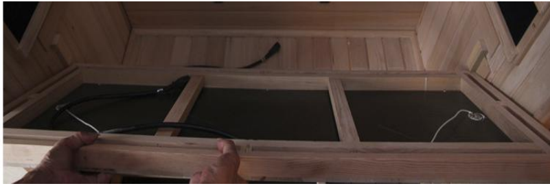
Figure 10 - Installing BENCH HEAT EMITTER PANEL
