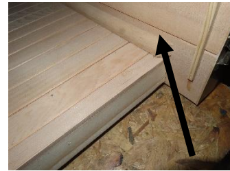
Trim molding of FRONT WALL PANEL resting on the FLOOR PANEL on the interior
