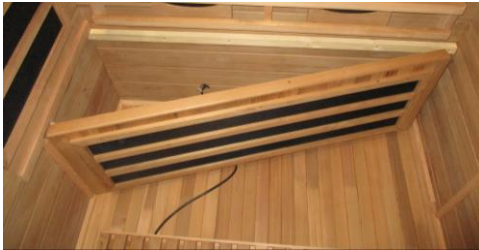
FIG-9 Installing Bench Heater
