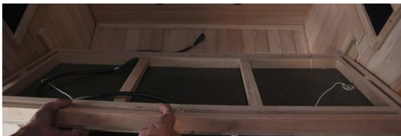
Figure 10 - Installing BENCH HEAT EMITTER PANEL
