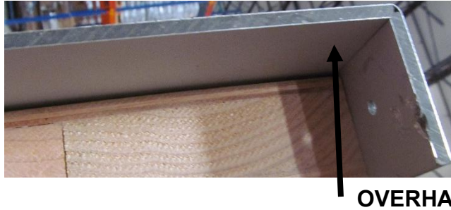
Front Section of the EXTERIOR ROOF PANEL with the OVERHANG
