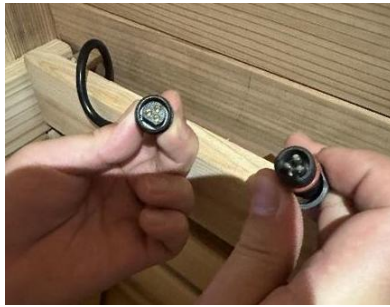
Heater Cord Connections
