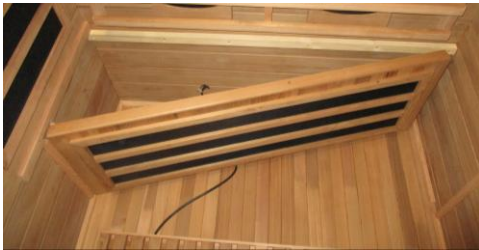
FIG-9 Installing Bench Heater
