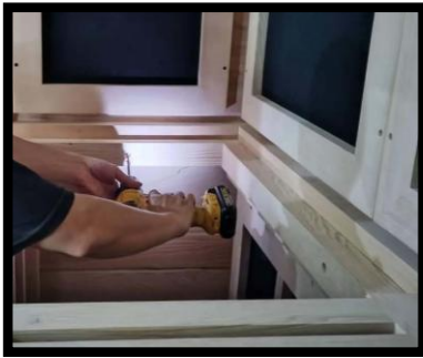
Screw to Side Panels Figure 13
