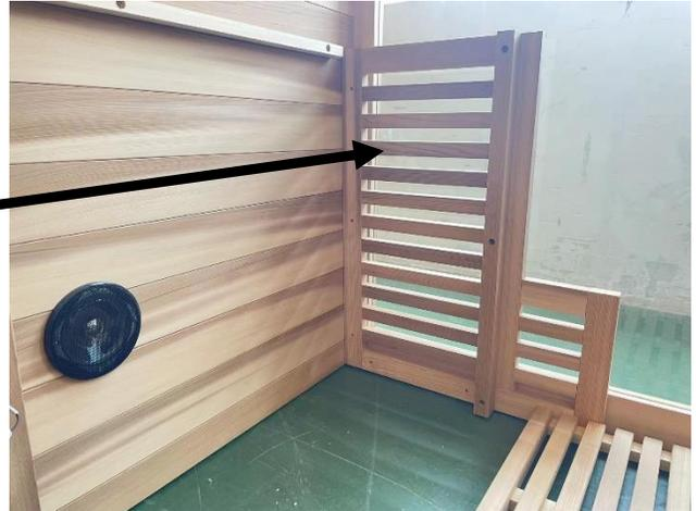
**BENCH SUPPORT PANEL will slide within the vertical slot on the SIDE BENCH SUPPORTS**
