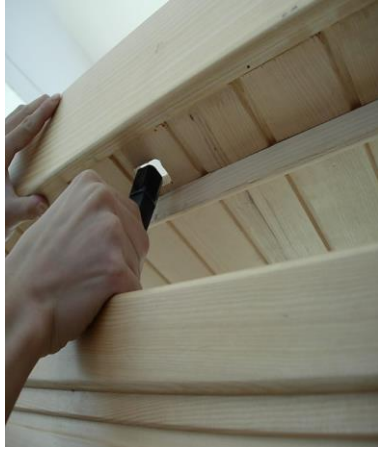
FIG-12 Slip cords/wires through corresponding holes
