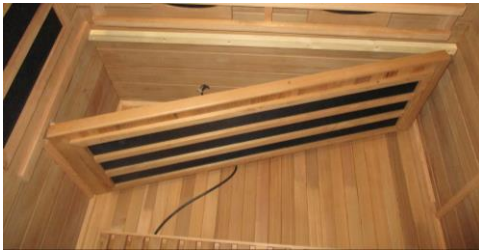
FIG-9 Installing Bench Heater
