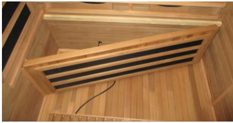
FIG-9 Installing Bench Heater
