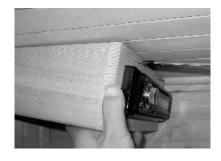
FIG-17 Screwing in the Radio Wood Housing
