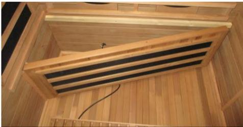
**FIG-9** Installing Bench Heater
