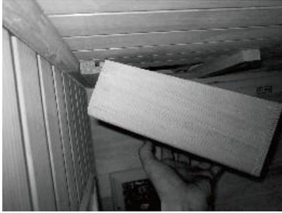
**FIG-16** Installing the Radio Wood Housing
