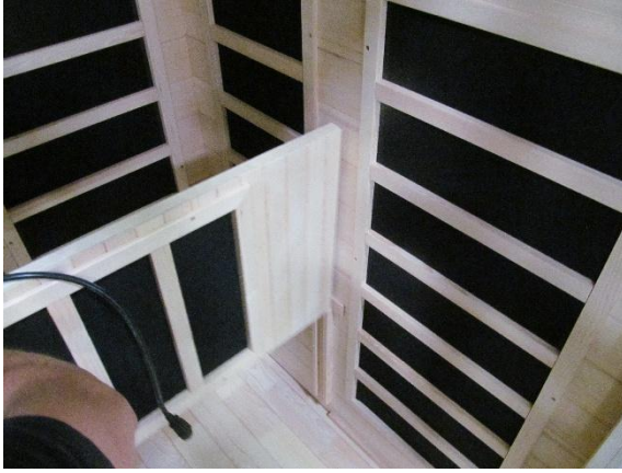
Installing the BENCH HEATER PANEL Figure 10
