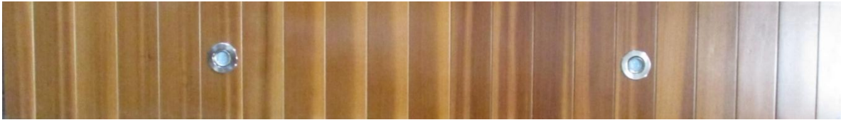
INTERIOR FRONT ROOF PANEL
