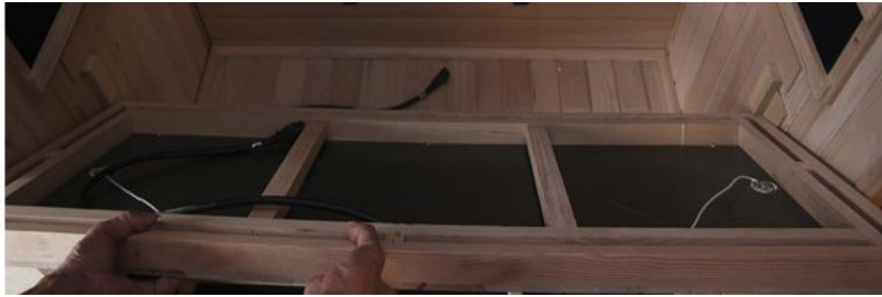
Figure 10 - Installing BENCH HEAT EMITTER PANEL
