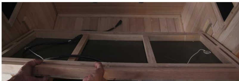
Figure 10 - Installing BENCH HEAT EMITTER PANEL
