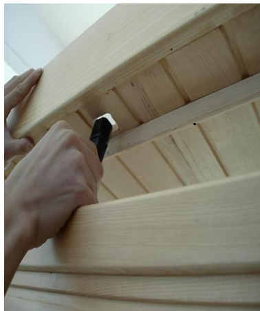
FIG-12 Slip cords/wires through corresponding holes
