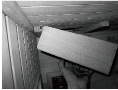
FIG-16 Installing the Radio Wood Housing
