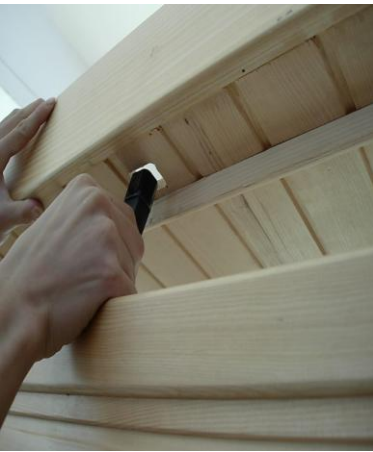
FIG-12 Slip cords/wires through corresponding holes
