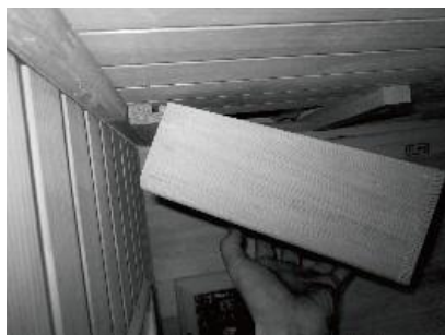
FIG-16 Installing the Radio Wood Housing
