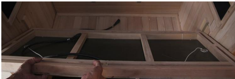
Figure 10 - Installing BENCH HEAT EMITTER PANEL
