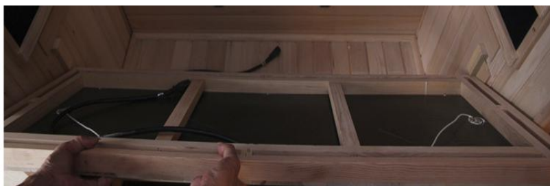
Figure 10 - Installing BENCH HEAT EMITTER PANEL
